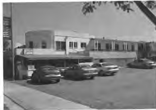
The on-site parking requirement contributes to the fragmented pattern of development in the Town Center.
